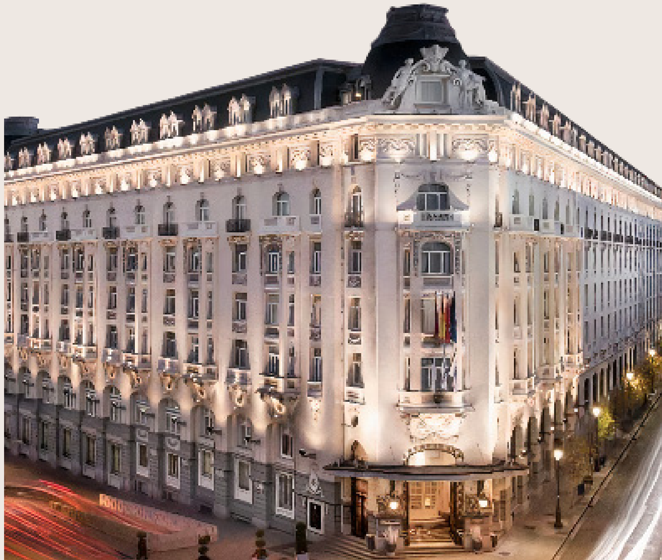
In 2023-24, Fernandez Molina will do a complete renovation of the Hotel Palace 5* Madrid
